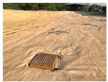
We designed a liner system using our poly urea product, AM1949. Additionally, concrete sections were added and placed on top of the earth and stone berm wall. This increased the capacity and allowed for better attachment of the liner system to stop any wind uplift. Our liner system proposal was reviewed by the engineering firm and submitted to the New York State DEC, who then gave approval. We started working on site and completed the entire installation of our liner system in one week.
